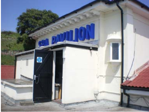
Roof area behind existing follow spot room
