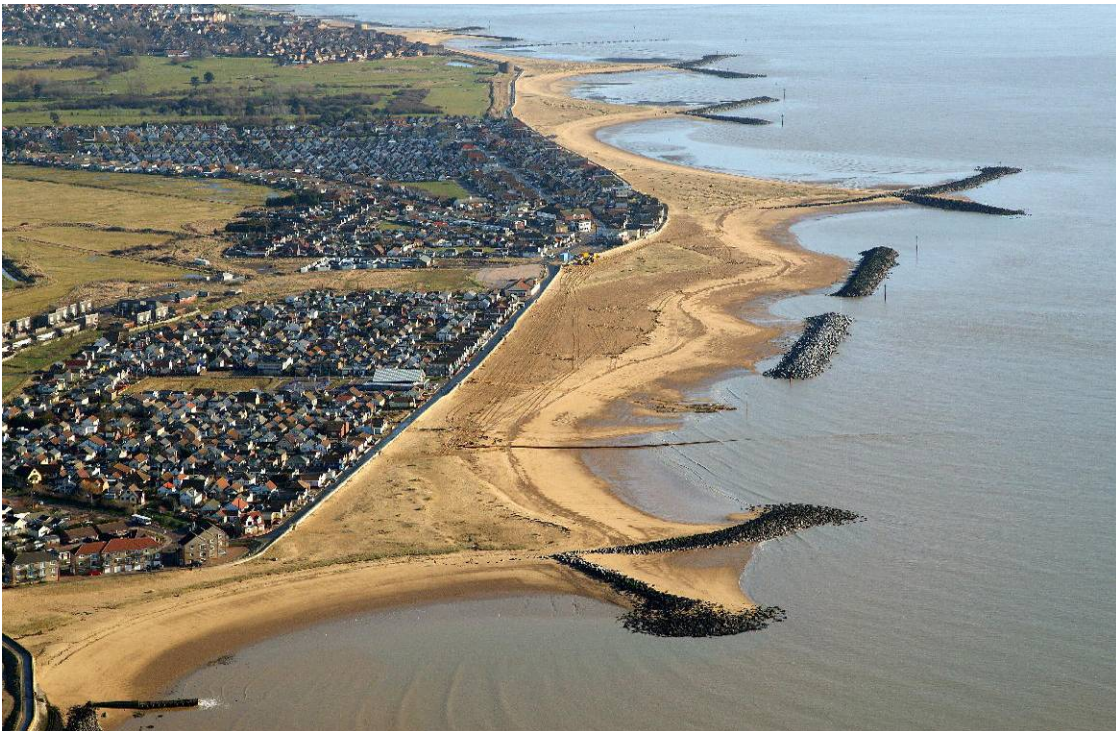
Figure 2-1 Coastal defences along the Tendring peninsula
