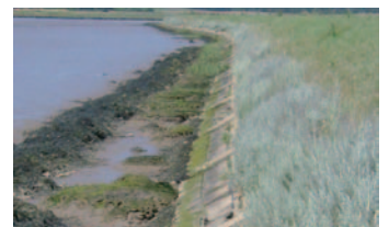
Concrete block revetment ④
