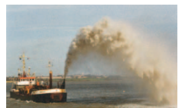
Foreshore recharge ②
