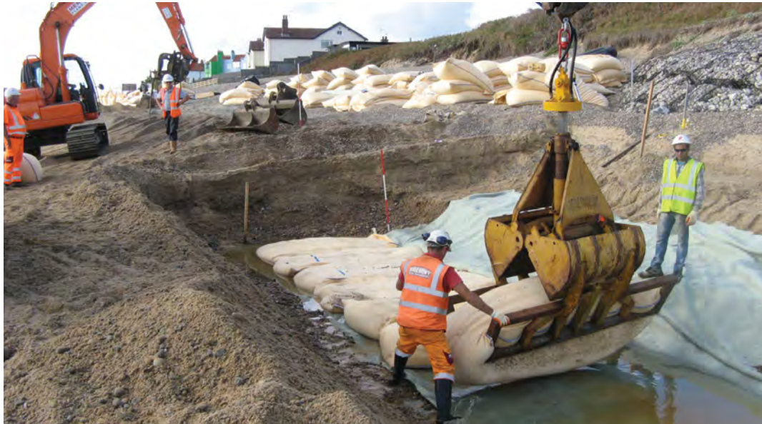
Work underway on putting in the bags at Thorpeness
