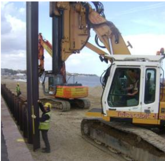
Steel sheet piling works
