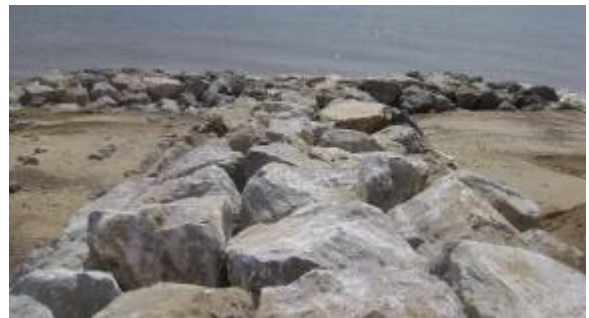
Completed fishtail groyne
