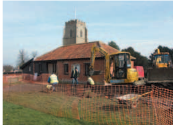
Work underway to improve access at Dennington
