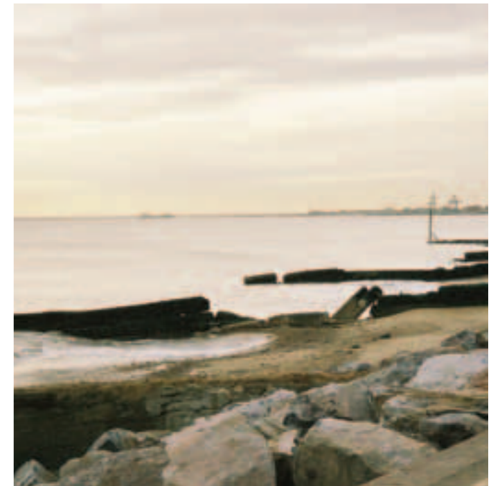
Have timber groynes had their day?
